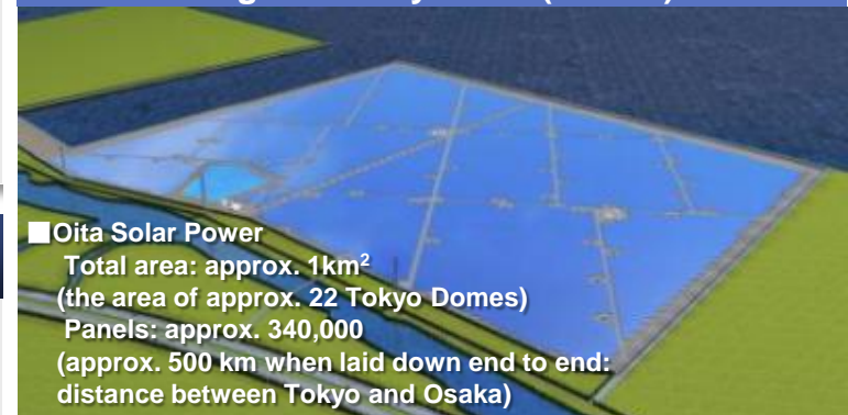
Japan's Largest class Mega-Solar Systems (82 MW)
